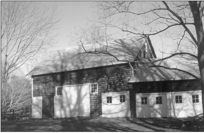
Photo 5. The extant c.1840 three-bay Anglicized Dutch barn in Montvale. In its original classic form the width of the nave was 18'-1" and the original side wall length was 30'-3".
