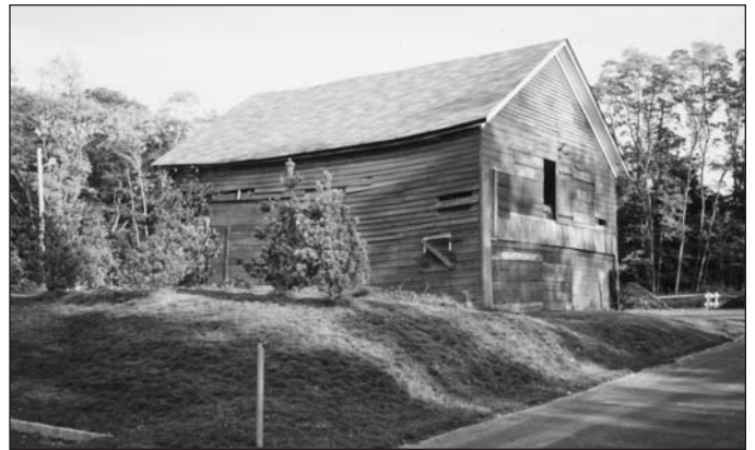
Photo 2. The now-raised Ackerman-Dewsnap Anglicized Dutch barn in Saddle River, New Jersey. This was originally a classic barn that was converted into a side wall entrance barn and only two of the original bays were retained. The barn was removed from its site about 1993 and its timbers were placed in storage.
