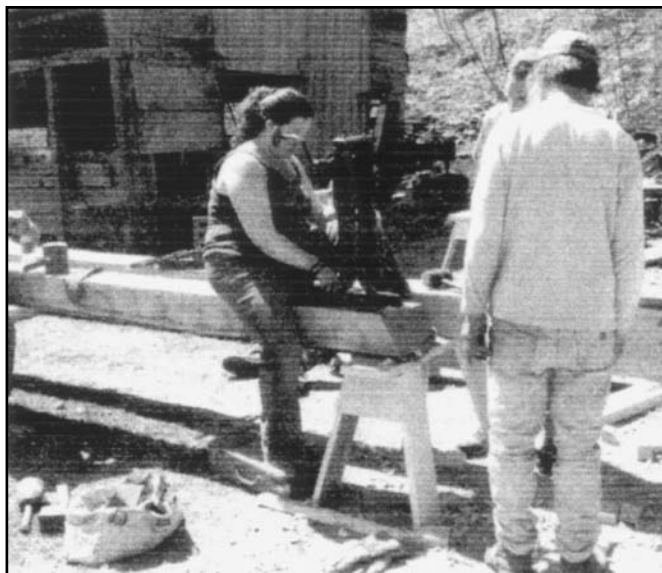
Boring holes by machine.
