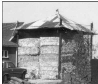
FIG 8 Barrack with steel roof and baled straw.
