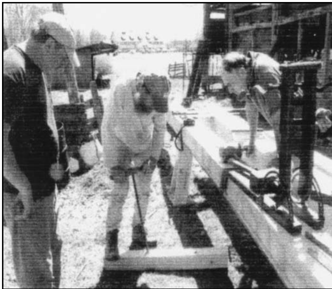
Boring holes by hand.
