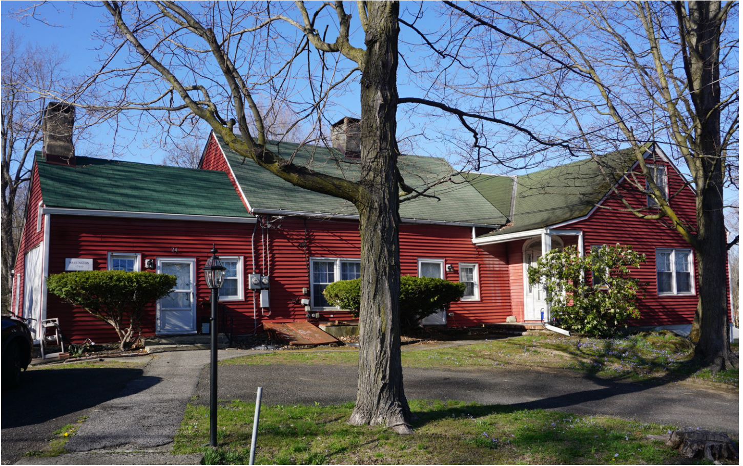
Fig.4: Micajah Lewis House, 24 Old Indian Rd., center section ca. 1750. Photo by John Ham, 2021.
