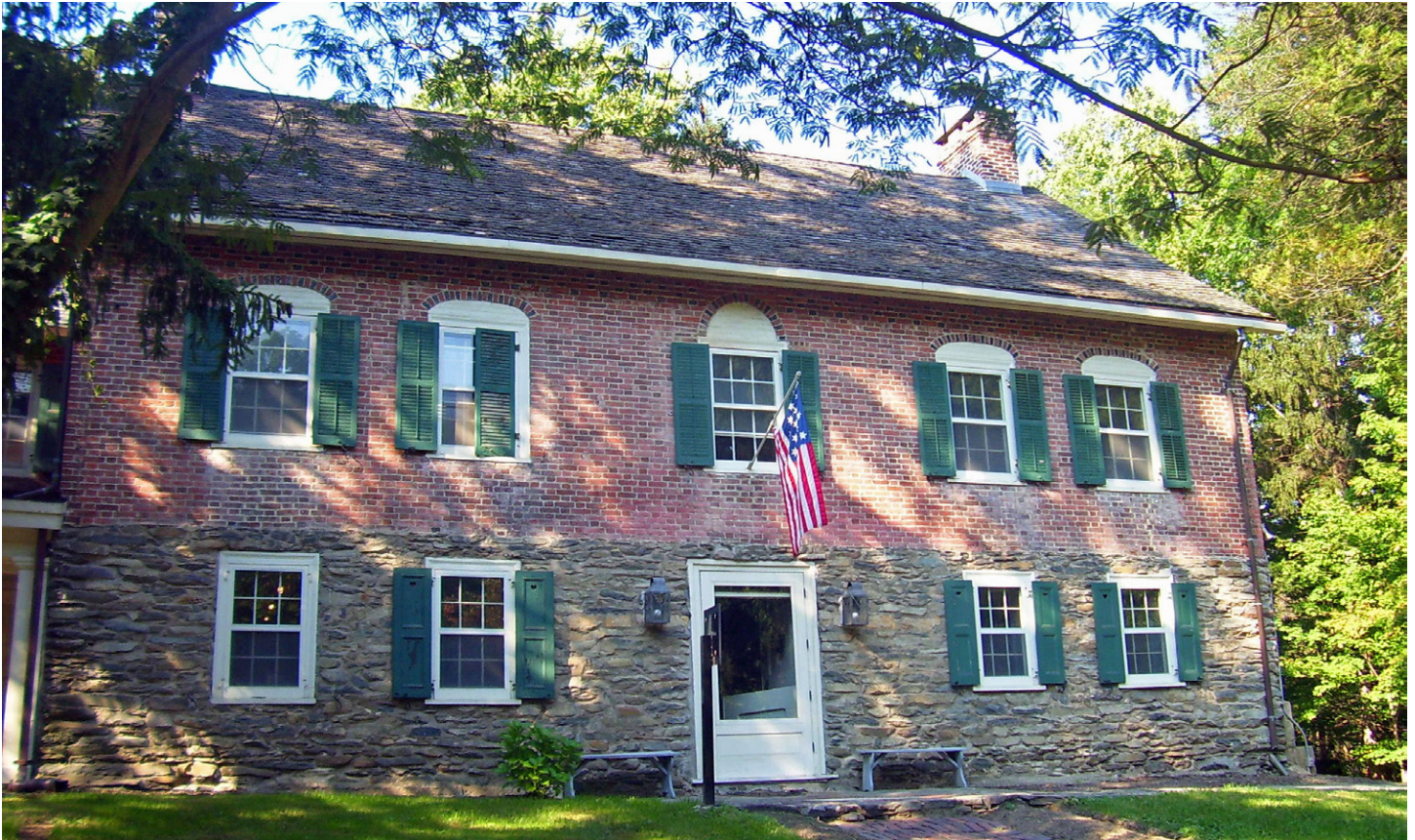
Fig.2: Gomez Mill House, Town of Newburgh, Orange County, ca. 1740. What likely was a wood frame upper story was replaced with brick by Wolfert Acker in 1772. Photo from Wikipedia.
