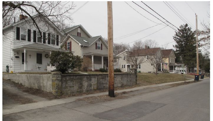
Figure 5. View north on west side of Oak Street showing 26, 30, 32-34 & 36 Oak St. left to right.
