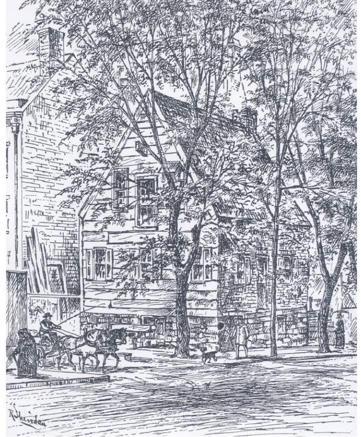
Fig.5: Engraved view by R. Sheridan, 1886. Although probably copied from the 1883 photograph, this image makes aspects of the building clear that are obscured in the earlier image. Among these are the intact hoist beam on the west gable end elevation and the door centered on the south elevation.
