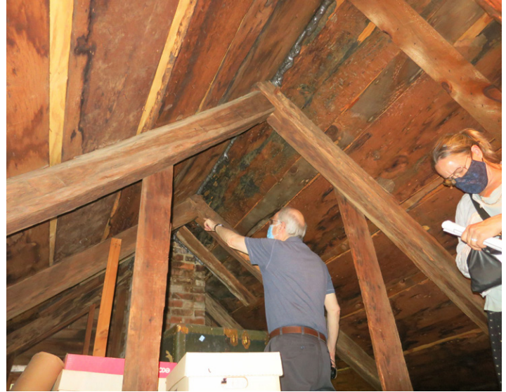
Roof framing, David Pratt House, 1777 Spencertown (June)
