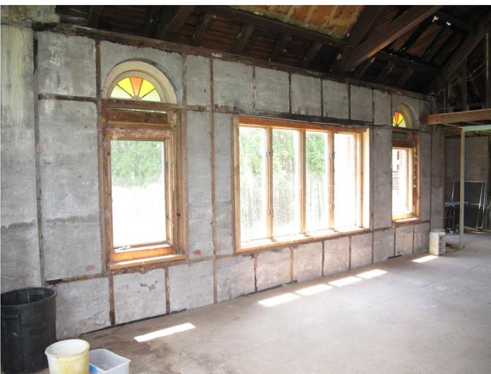
Fig.9: Great room, west wall showing loss of plaster, lath and studs embedded in concrete wall, 2021. Photo by Neil Larson.
