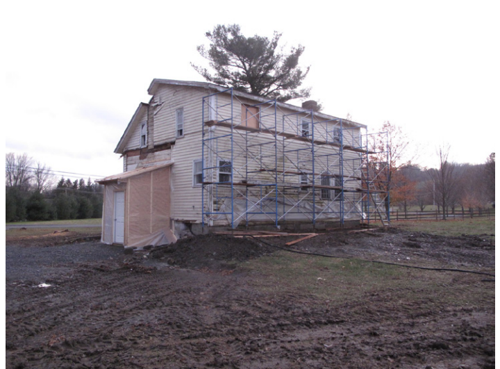
Fig.1: View from SW. The window to the right of the door originated as a second entrance. The double window on the west end replaced a doorway linking the house to a previous wing; windows in the upper story of the front façade are mid-19th-century additions. Photos by W. R. Wheeler, 2019.
