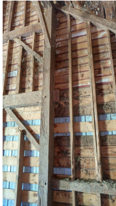
Fig. 3: North wall bent, with two anchorbeams. Photo by John Cannon.
