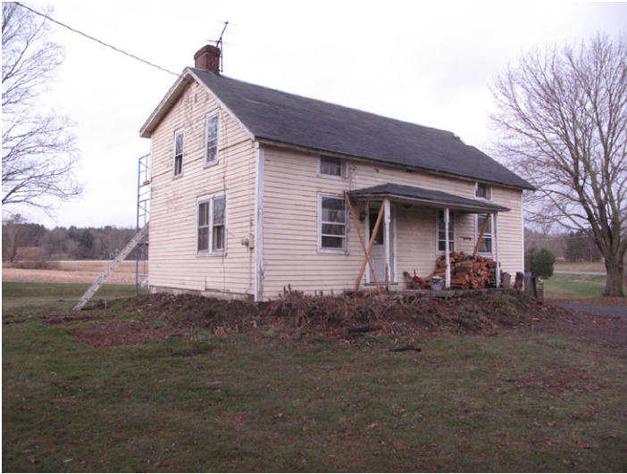
Fig.1: View from SW. The window to the right of the door originated as a second entrance. The double window on the west end replaced a doorway linking the house to a previous wing; windows in the upper story of the front façade are mid-19th-century additions. Photos by W. R. Wheeler, 2019.
