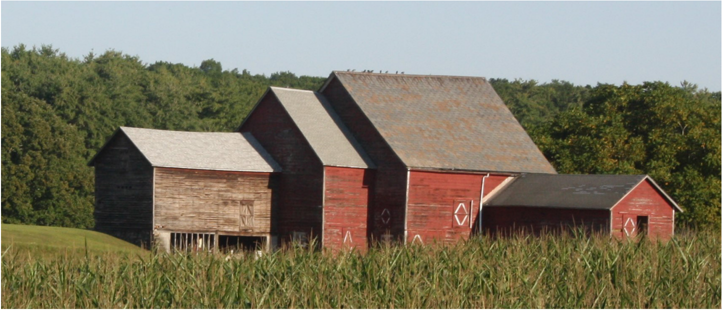
Fig.2: Eldred barn as seen looking west from Greene County Route 51, Town of Coxsackie. The original Dutch barn has the highest roof line. The cow barn addition is perpendicular to the rest of the structure. Photo by Ted Hilscher.
