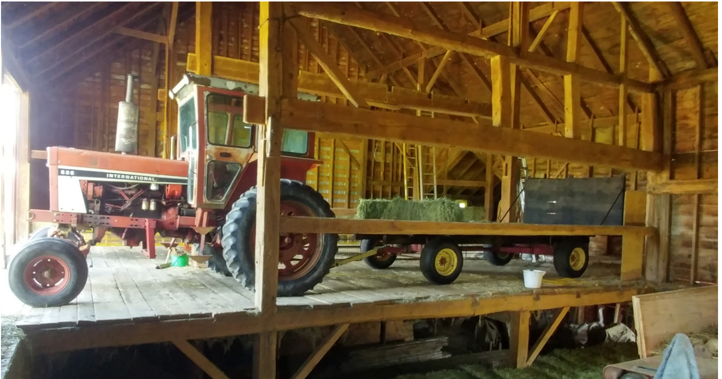
Fig.1: Interior of Eldred barn indicating H bents. Far wall is north wall. Photo by John Cannon.
