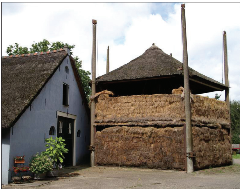
Figure 3. Four-pole hooiberg with pulleys at Franschepad, Blaricum, Netherlands. Photo Courtesy Gerard Grootveld.
