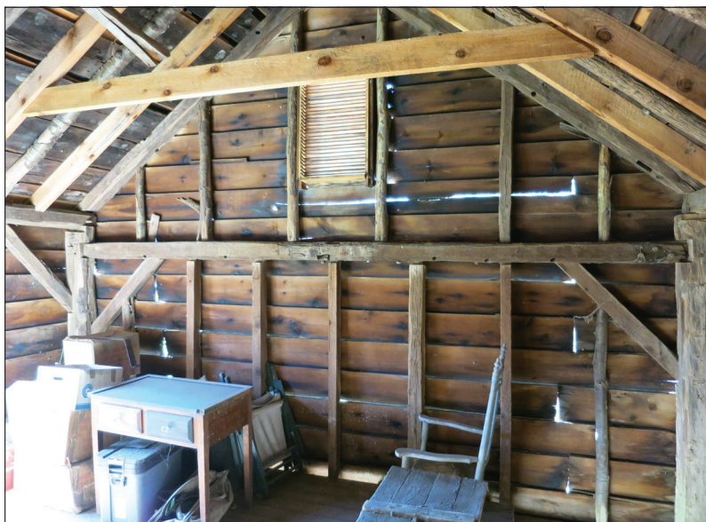
Figure 17. Interior of the Smith barn, showing barrack parts reused as rafters and dropped tie beam (Photo by author). The mortises in the pieces used as rafters may be for a raised platform.
