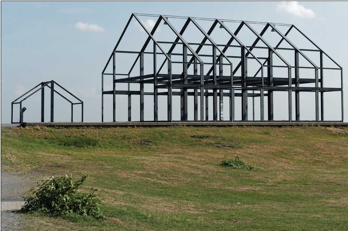
“Hallenhaus auf der Halde” in Neukirchen-Vluyn in northern Germany. Constructed in 2014, based upon drawings of the Deertz barn in Schoharie County by Malcolm Kirk. A project of WES & Partner of Hamburg and Observatorium of Rotterdam (Photo by Arnoldius, Wikimedia Commons 2016).
