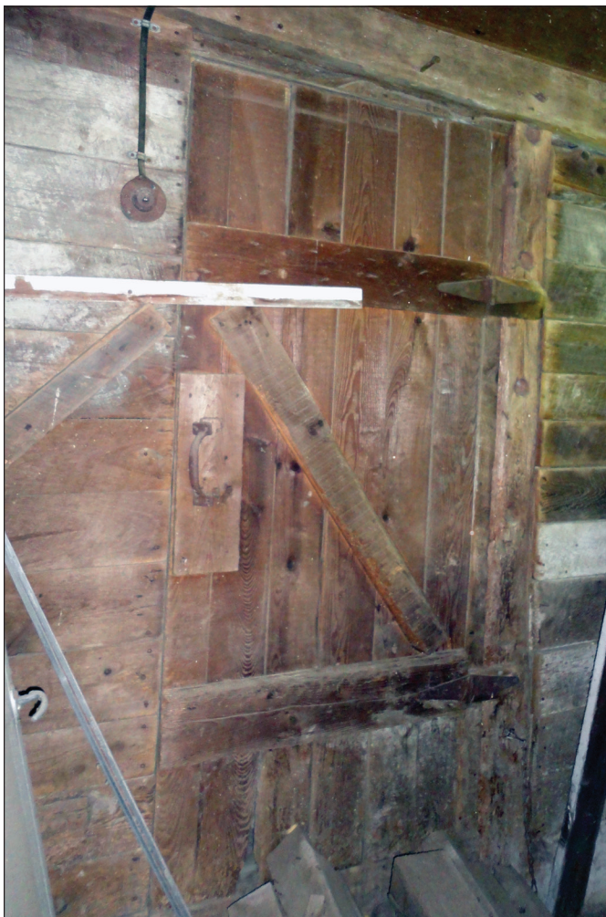
Figure 19. Door with its right hand jamb fabricated from a reused barracks part in the Muia barn, Altamont (Photo by author).
