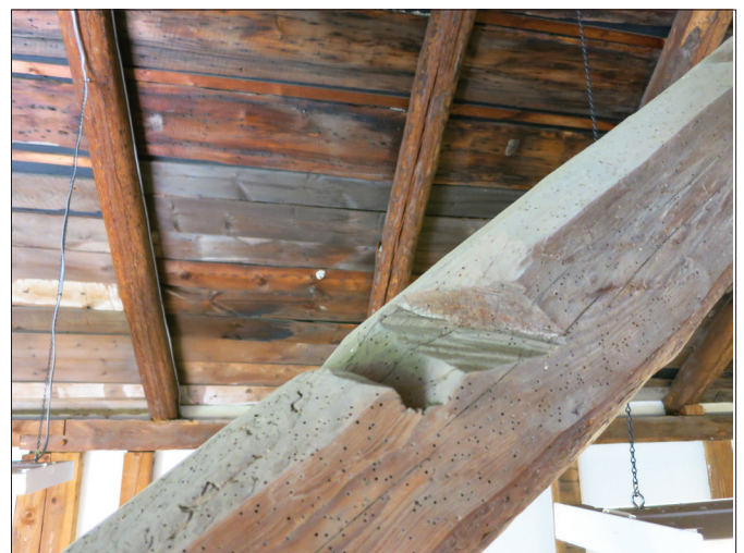
Figure 16. Detail of one of the reused plates in the Embought Road barn, showing a typical notch (Photo by author).
