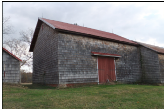
Photo 2. The Smock Dutch-Anglo eave-wall entry barn on Longbridge Road in Holmdel is on a township owned property. The barn, in excellent condition, was built c.1820 or 1830 (Photo by Greg Huber).
