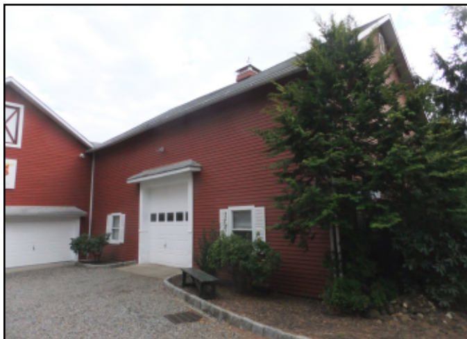
Photo 17. The Smock barn on Hillsdale Road in Colt's Neck is a previously unknown eave-wall entry barn type. The layout of its H-bents suggests a construction date of c. 1800 (Photo by Greg Huber).
