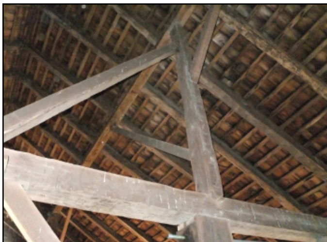
Photo 3. The Stevenson Dutch-Anglo Barn on Vanderburg Road in Marlboro; this barn illustrates the use of two levels of purlin plates in eave-wall entry barns. The vertical queen post supporting the "Anglo" purlin plates is supported by the "Dutch" purlin plate seen at the bottom of the photo (Photo by Greg Huber).
