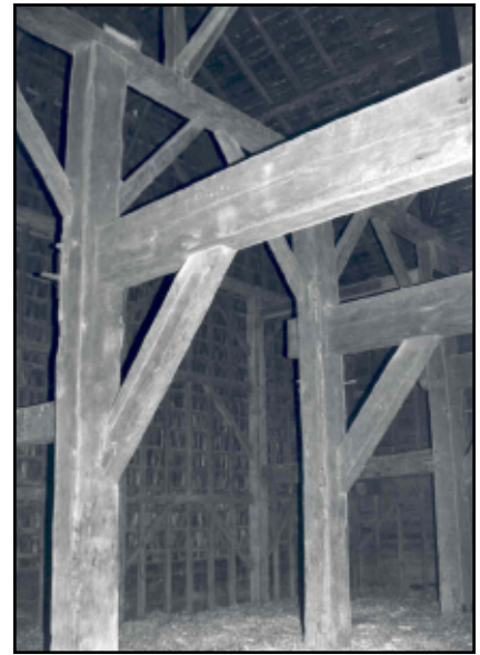
Photo 8. A second view of the Schenck Americanized barn, the "Mammoth in Monmouth County", with view of part of three inner H-frames. One H-frame post was over 20 inches in width, making it the largest post in any Dutch related barn known to this author. Inner anchorbeams were each over 20 inches in height (Photo by Gail Hunton).
