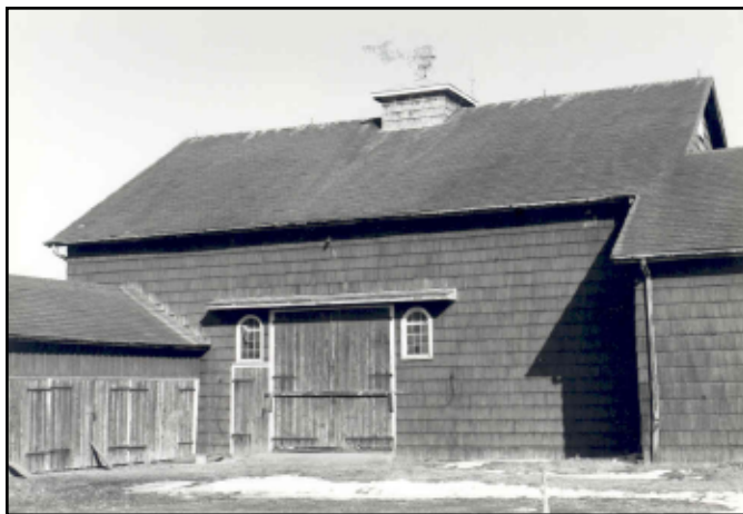
Photo 7. The Schenck Americanized eave-wall entry barn on Holmdel Road in Holmdel. This structure had the largest timbers the author has seen among Dutch related barns in either New York or New Jersey. The middle bay with its H-frames was part of three-aisle barn built circa 1780; the barn was converted c. 1850. It was lost in a fire in the fall of 1998 (Photo by Gail Hunton).
