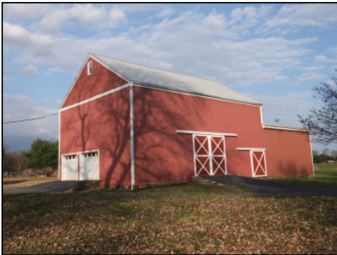
Photo 1. The Stevenson Dutch-Anglo barn on Vanderburg Road in Marlboro is an original condition eave-wall entry barn. The exterior walls are covered with modern materials. Barn built about 1830 (Photo by Greg Huber).
