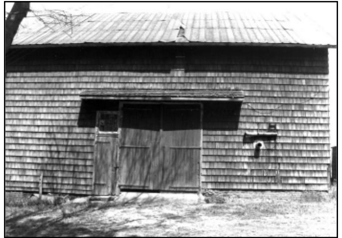
Photo 13. The Smock Dutch-Anglo barn; a close-up view of the sidewall wagon doors with flanking human door at the left side. The barn has a pentice roof projection that protects the doors from the weather (Photo by Gail Hunton).
