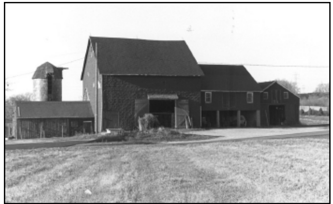
Photo 4. The Schanck Anglicized barn on Conover Road in Marlboro. This barn has the largest inner bent anchor-beams of any Dutch related barn seen by the author in either New York or New Jersey, one being just shy of 25 inches. The original three-aisle barn was built about 1790 to 1800 and was converted c. 1850 (Photo by Gail Hunton).
