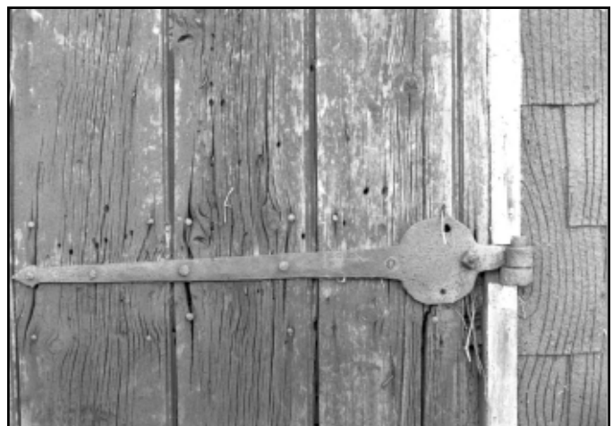
Photo 5. Classic Dutch-style hinge with pancake disk at the proximal end of hinge. Pad hinges such as that seen here were used throughout the Dutch-American settled areas (Photo by Gail Hunton).
