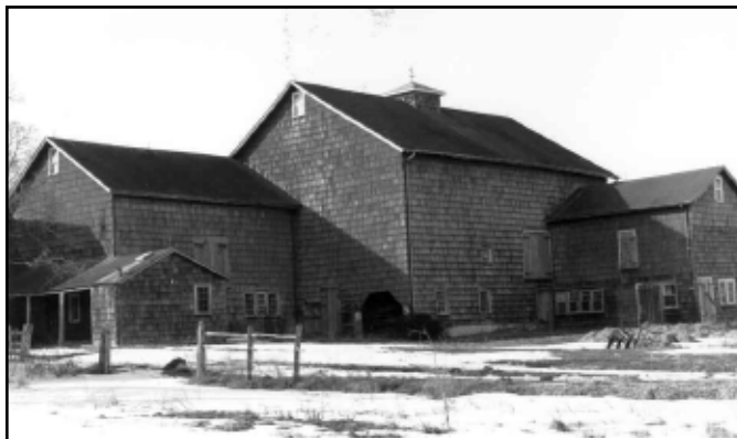
Photo 6. Array of barn structures at the Schenck homestead. Main Americanized barn with basement is seen in the middle; frame additions at each side (Photo by Gail Hunton).
