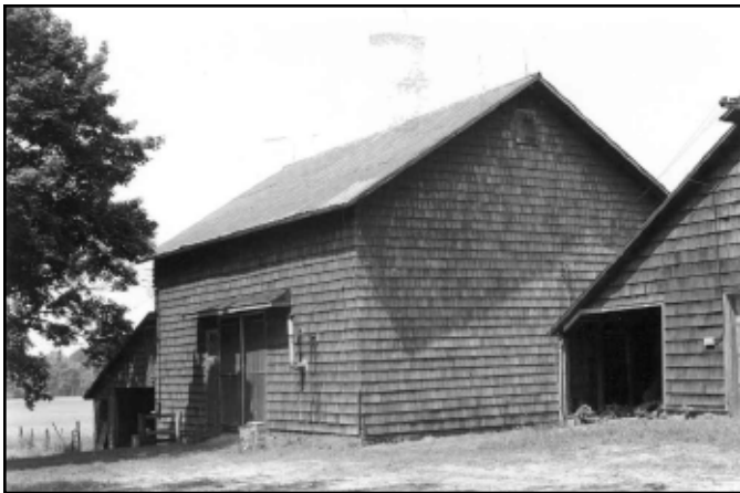
Photo 12. The Smock Dutch-Anglo eave-wall entry barn. Framed farm structures appear at each side of the main barn (Photo by Gail Hunton).
