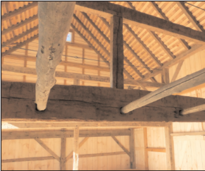
Photo 7. The back side of the swing-beam in the ground barn in Cranbury, Middlesex County, New Jersey includes widely spaced mow poles to support farm crops in end bay.
