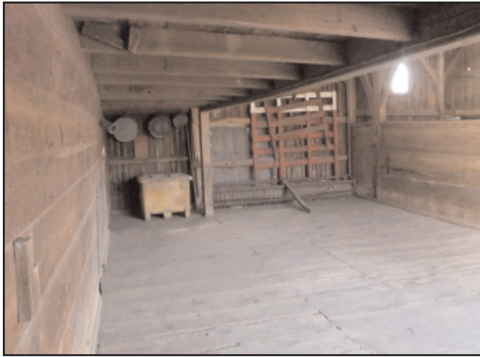
Photo 9. Swing-beam and almost seven foot wide alcove area in an Exeter Township, Berks County Standard barn dated 1805. The beam left clear a wide area for threshing and a turnaround area for animals attached to wagons.
