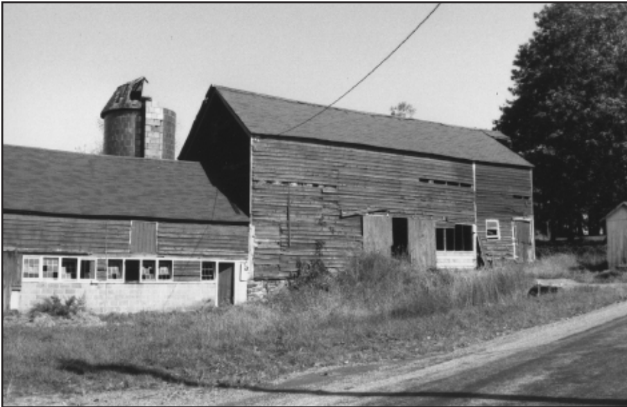
Photo 3. Exterior view of the side-wall wagon-entry swing-beam barn in Bethlehem Township, Warren County, New Jersey. Note the one-bay addition of the barn at the right.
