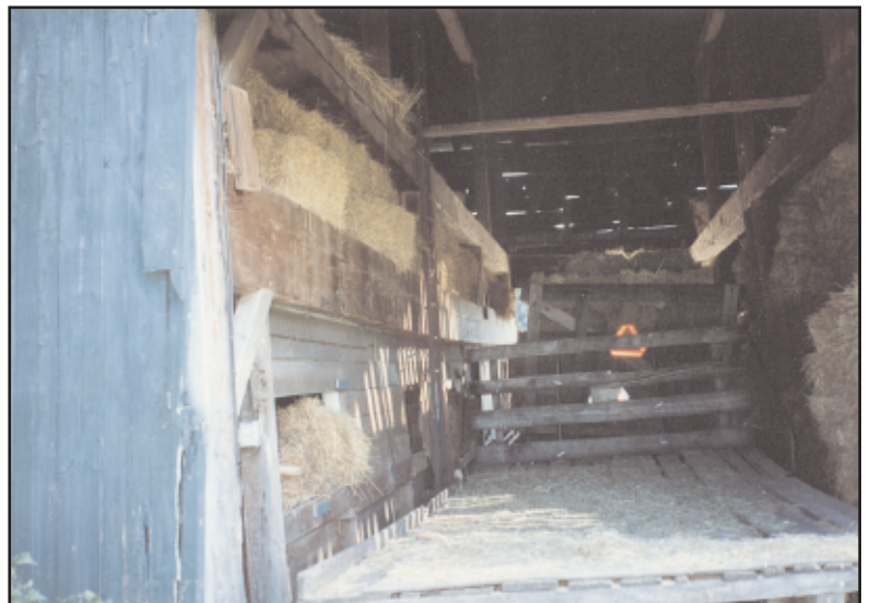
Photo 12. Interior view of Barber barn, showing massive 50+ foot long swing-beam.
