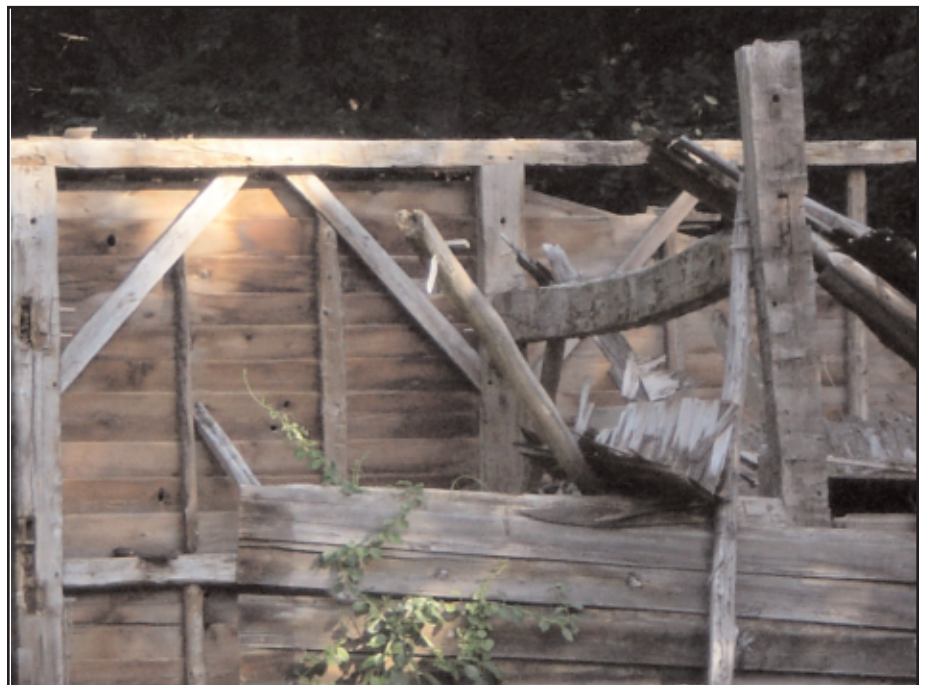
Photo 3. Detail of barn, showing anchorbeam, August 2009.
