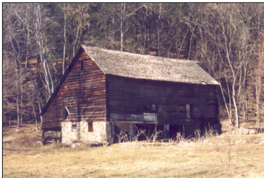
Photo 1. The LeFevre barn in April 2003. Wood roof shingles are plainly seen along with horizontal weather-boarding. At left on the basement level is the recess which initially suggested a possible connection to Pennsylvania fore-bay barns.
