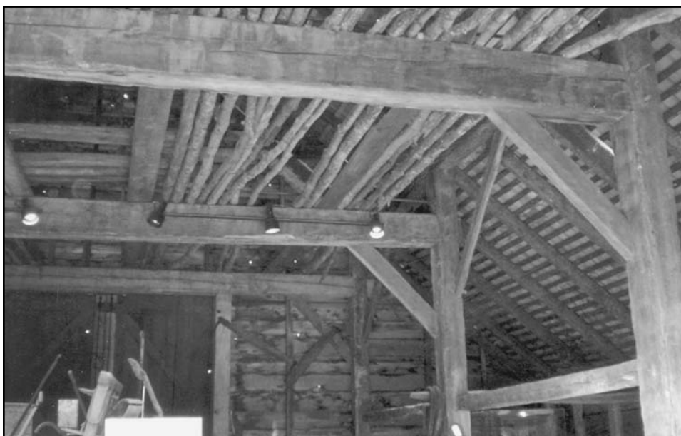
Photo 2. Interior of the Wortendyke barn, a good example of three traits that are often found in Bergen County barns. These traits include short verdiepinghen , purlin braces connected to H-frame posts two feet below the anchorbeams, and low side walls.
