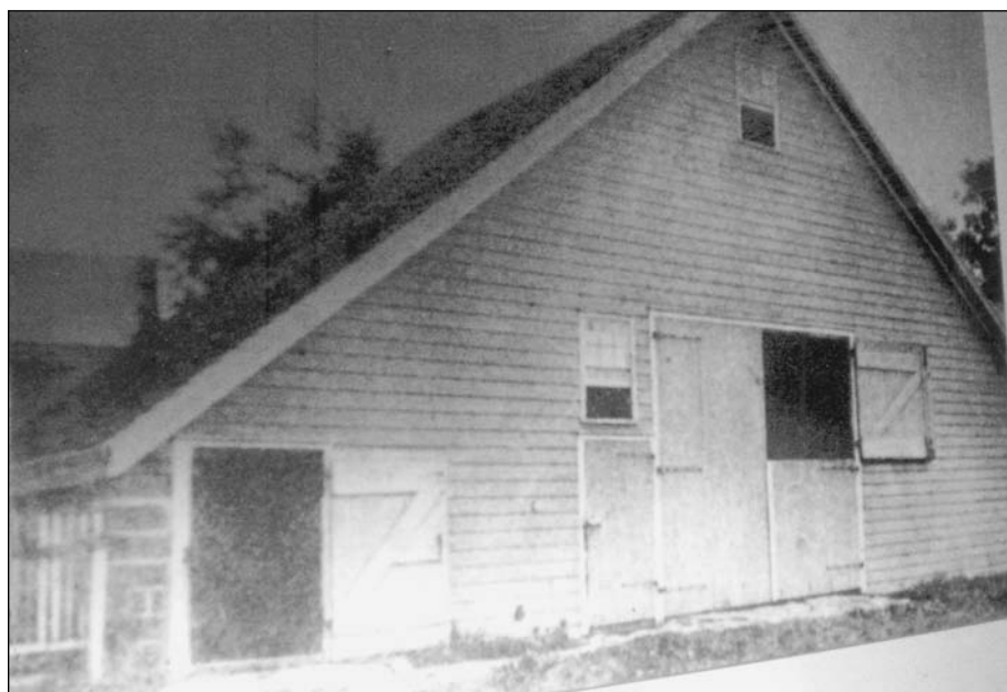
Photo 4. The 18th-century Zabriskie three-aisle barn in Paramus, New Jersey has low side walls and a relatively high peak, creating outstanding proportions. Note side wall at left with stone construction.
