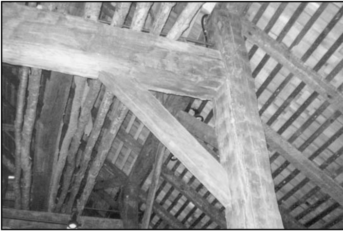
Photo 3. Interior of the Wortendyke barn. This barn has extremely short verdiepingh of only 22 inch length, which apparently precluded inclusion of raising holes.
