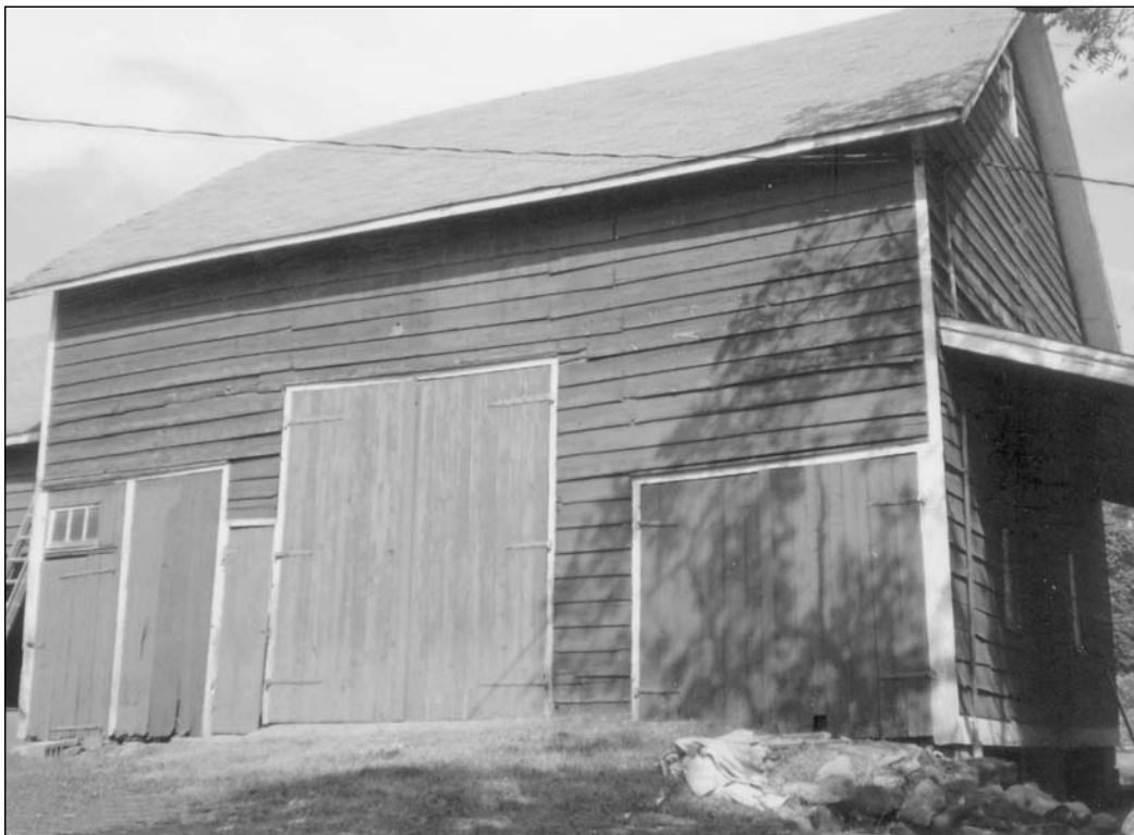
Photo 8. The George Demarest Americanized Dutch barn in Hillsdale, New Jersey is the only Dutch barn in Bergen County that includes a basement. The original three-aisle barn was likely erected before 1800. The inclusion of both the side wall wagon entry and the basement may have taken place at the same time.
