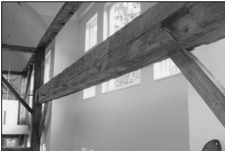
Photo 9. The Durie-Belcher Anglicized three-bay Dutch barn in Haworth, New Jersey was recently moved about one hundred feet from its original location and converted into a residence. The original three-aisle barn was likely constructed before the Revolution. Later it took a second three-aisle form and still later a barn with a side wall wagon entry. Thus to date it has had four barn lives.
