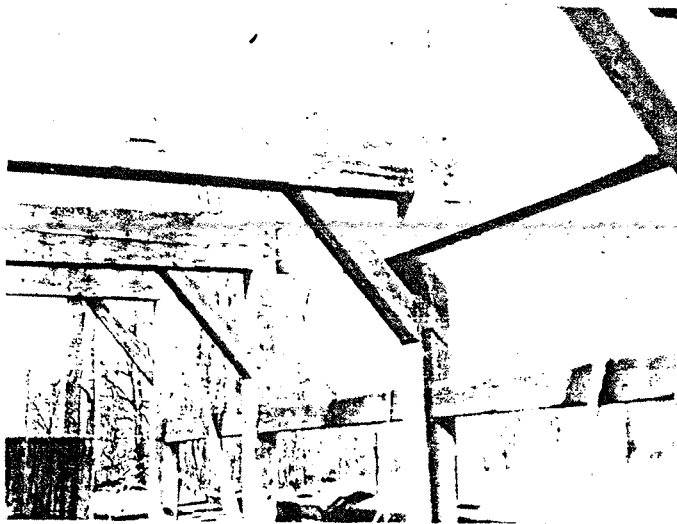
Anchor Beams of Wemp Barn before they were lowered
