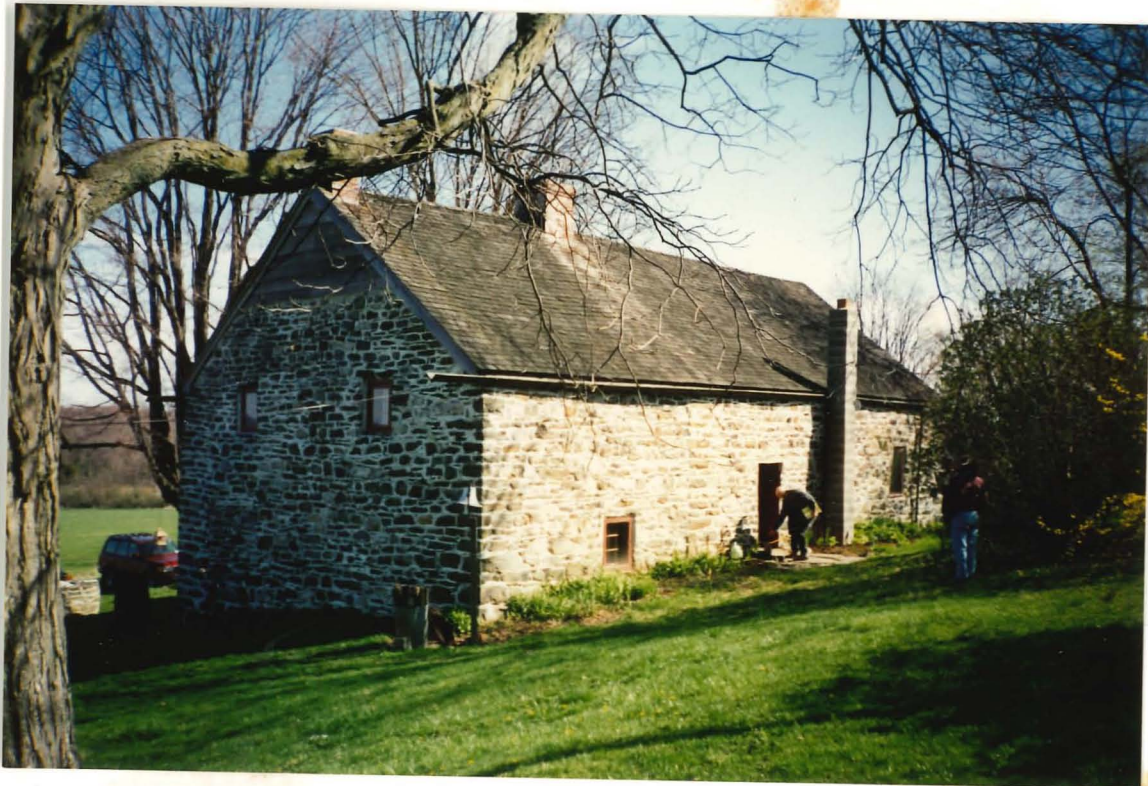
Photograph 1. Back of the Terwilliger/Coomer stone house, by John Stevens
