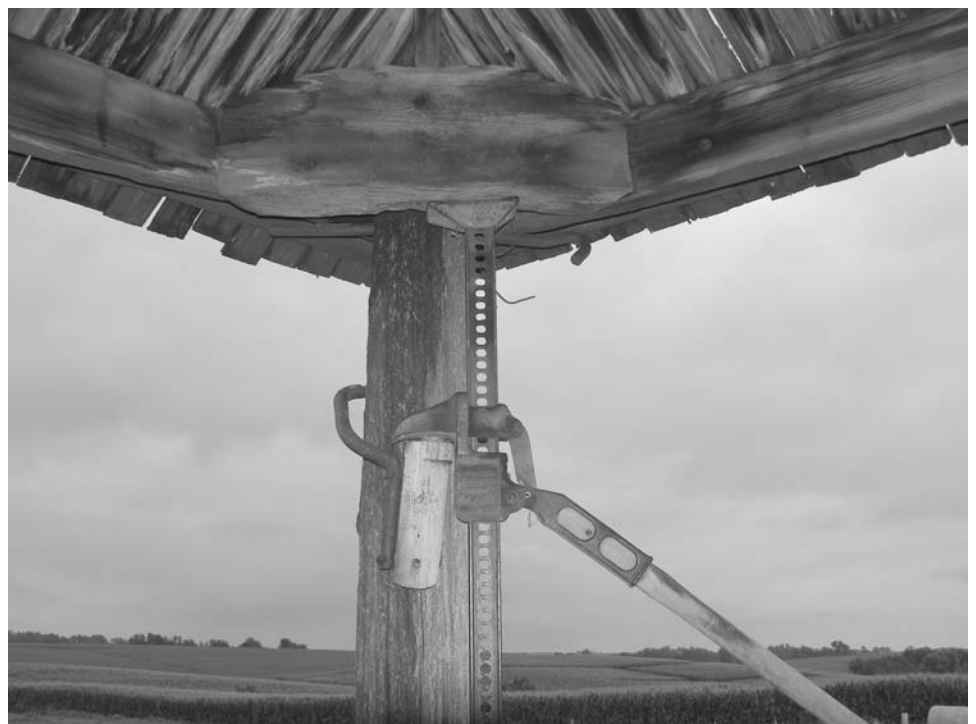
Photo 2. Corner detail showing roof jig in place.
