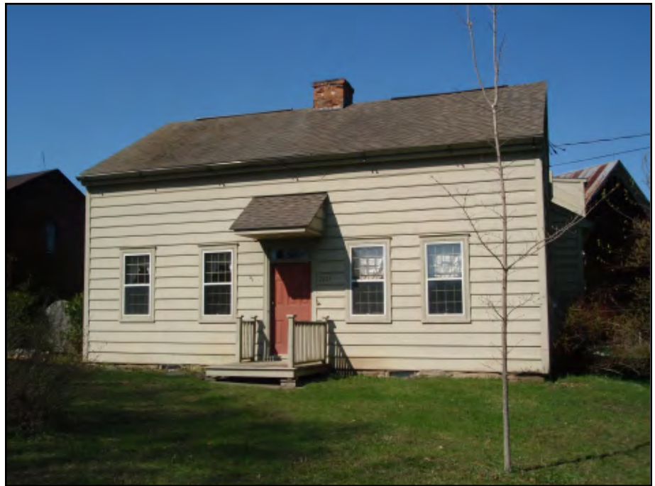
Photo 2. View of the Dockstader house, looking north-northwest.
