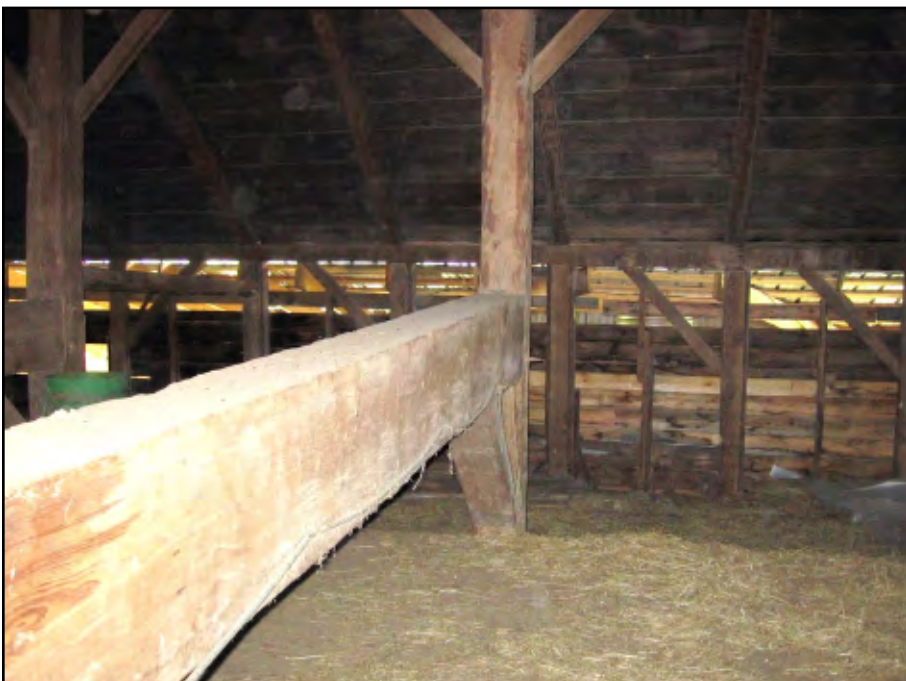
Photo 4. View showing the wall braces.
