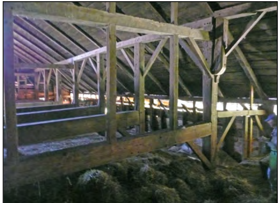
Photo 2. The original six bays of the Pindar barn, showing the join with the newer section at right.
