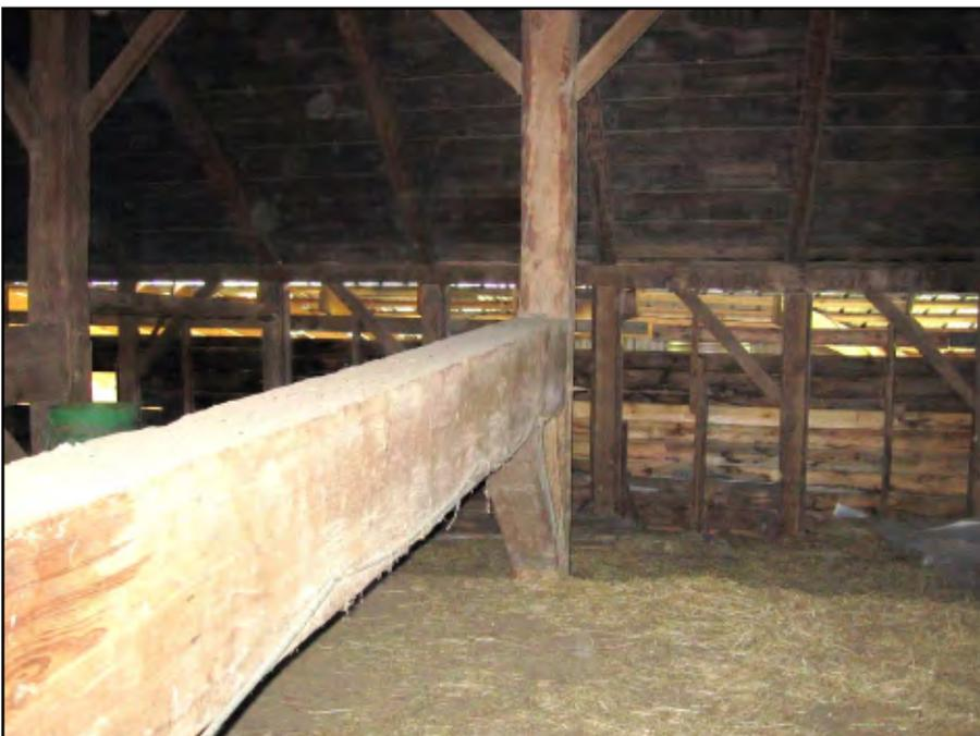
Photo 4. View showing the wall braces.
