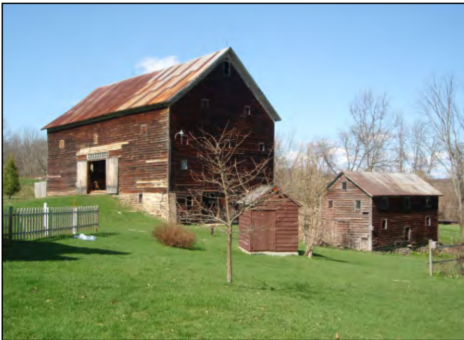
Photo 1. View of the Dockstader-Bergen barn, looking northwest. The smokehouse can be seen in the foreground; a small barn used for horses and chickens to the right (all photos taken by the author in April 2010).
