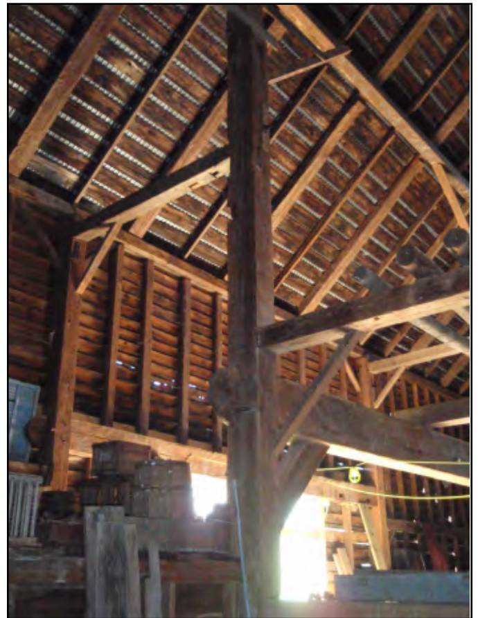
Photo 5. Interior of the Dockstader-Bergen barn, looking southwest showing bents 1 and 2.
