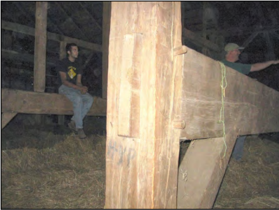
Photo 3. Detail of end of a typical anchorbeam-post connection at bent VI. Kim Balfour is seen at right; the owner's son sits on the anchorbeam of bent VII.
