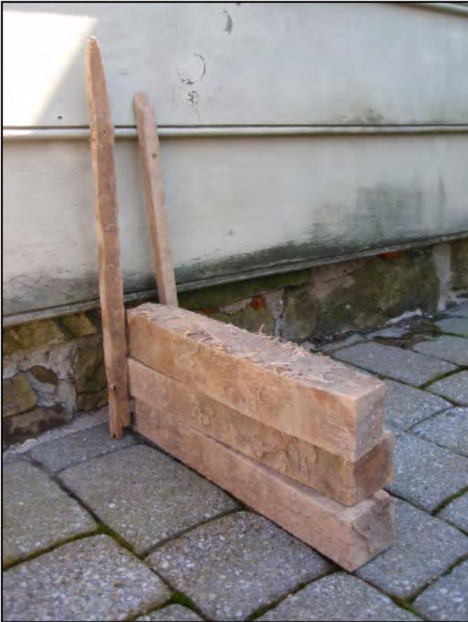
Photo 4. Some of the components of the wall infill. Mud and grass was packed around each of the horizontals which spanned between the bent posts of the house.
