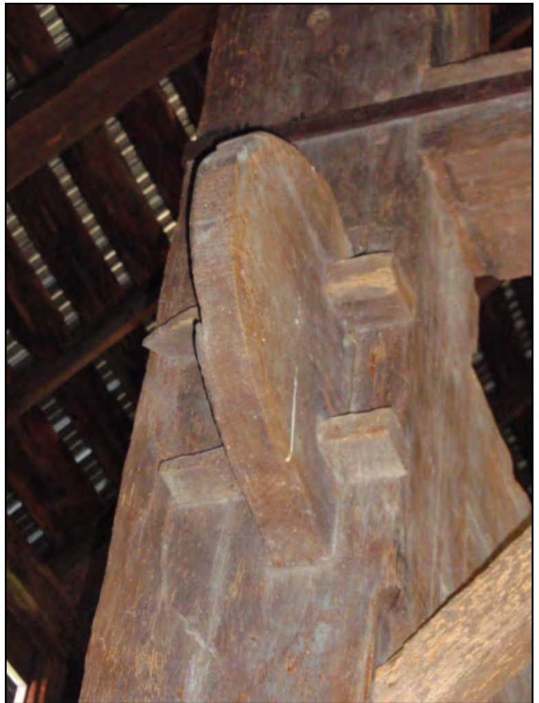
Photo 6. Detail of the east end of bent 2 showing the paired wedges.
